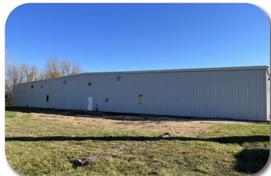
WEST SIDE OF BUILDING
