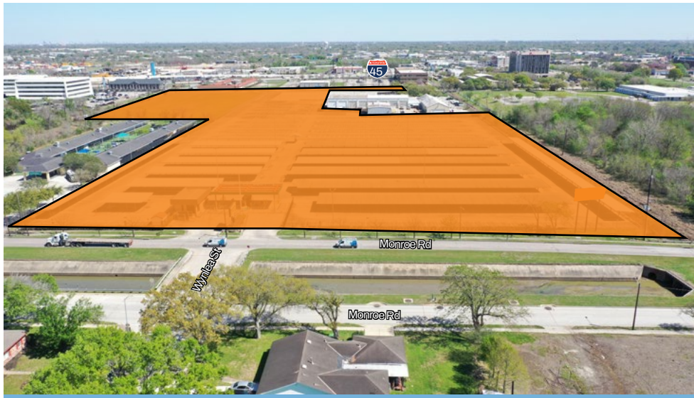
PROPERTY FACING EAST
