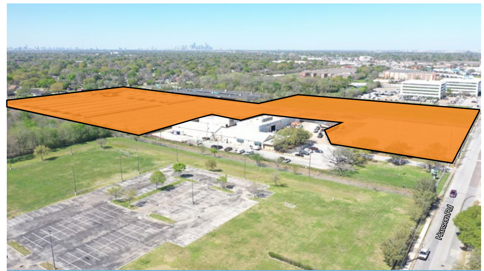
PROPERTY FACING NORTH WEST
